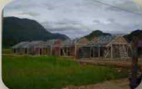
ADB House Banda Aceh
